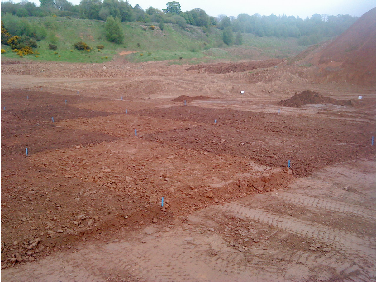
Plate 1 – Placed Material in Trial Pits
